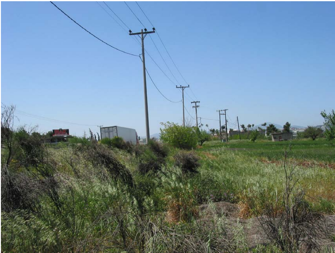
Figure 1. The location where the fire started, next to the National Road 1. Some burned shrubs are seen in the foreground. The electric power transformer suspected for causing the fire is visible at a distance in the middle of the photo.
