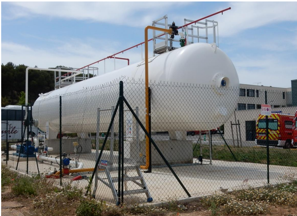
Figure 14. The pressurized tank providing fuel for the “simulated burning forest”
