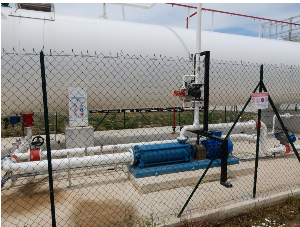
Figure 15. The piping/pumping system for distributing the propane to the “forest”
